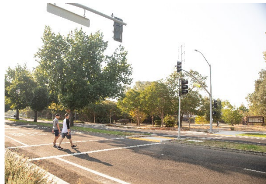
Figure 24. Signalized pedestrian crossing in Elk Grove
